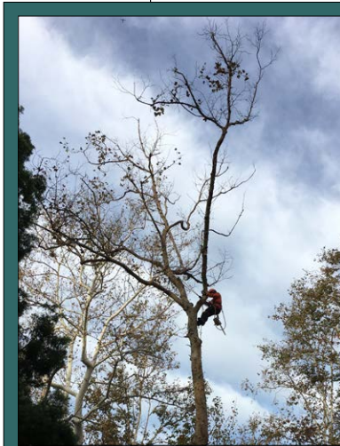
A worker removes top branches from a dead tree in the Main Green. The tree will be gone by the end of the day.
