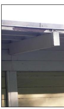
Roof framing components at many garage structures have areas of deterioration or failure, as seen in two separate locations in the above photos.
