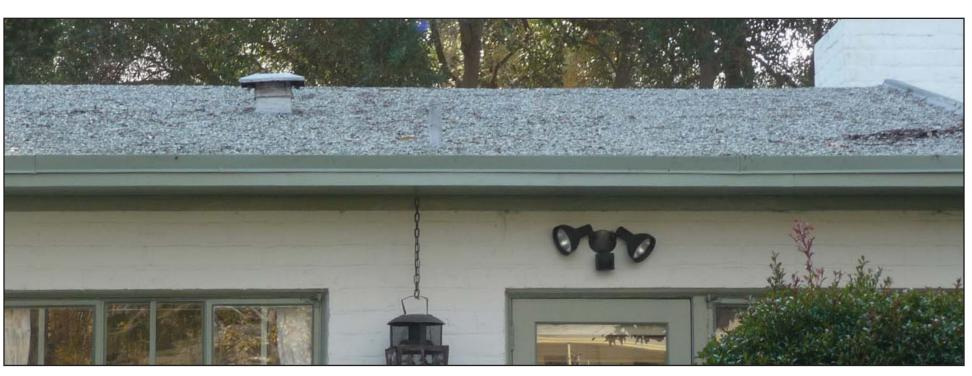
Built-up roofing with small gravel ballast, seen above at Building 48, can be found at the roofs of all residential buildings.
