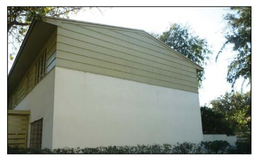
Stucco finish and horizontal wood siding of shiplap construction
